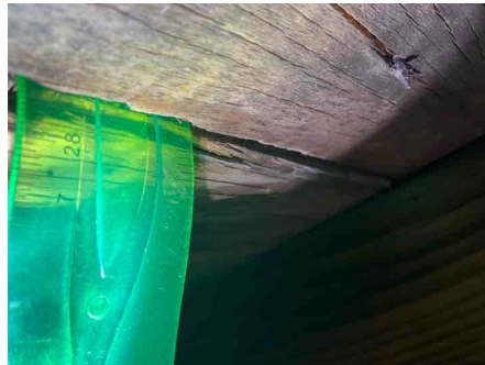
1/2 inch thick sheathing
